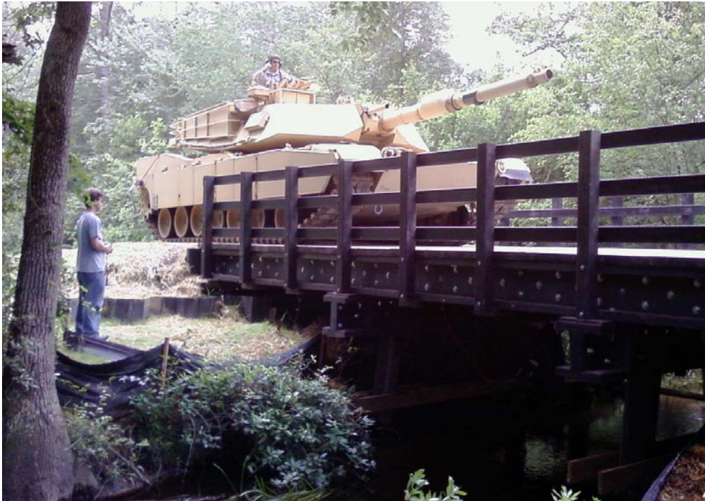
Figure 6. M-1 tank crossing the thermoplastic composite bridge during initial load testing
