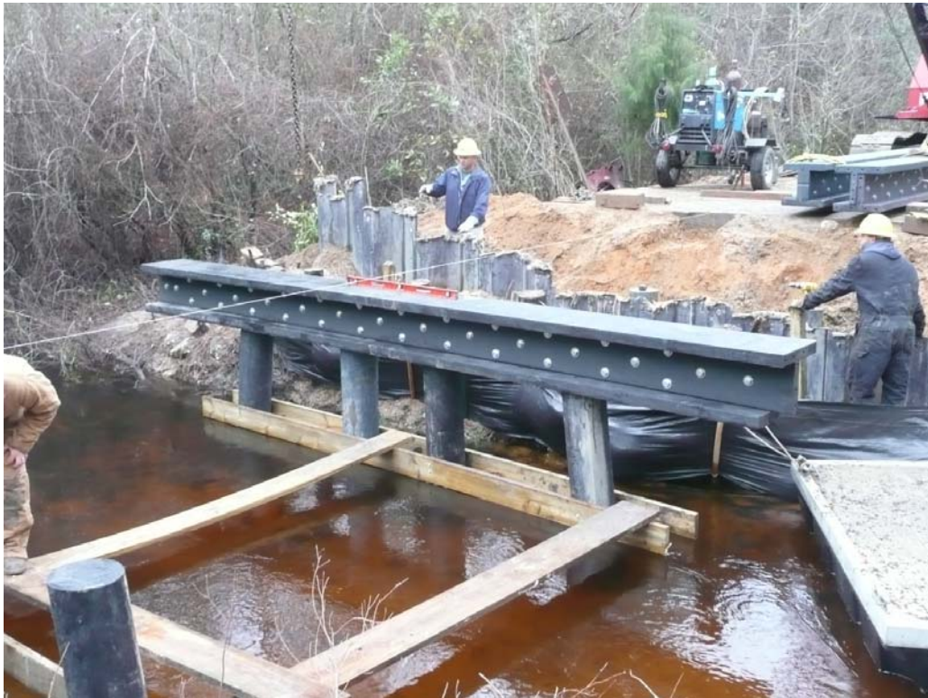
Figure 5. Construction of thermoplastic composite I-beam bridge at Fort Bragg.
