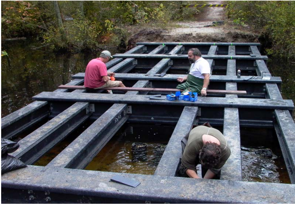
Figure 3. I-beam designed bridge being constructed at Wharton State Forest, NJ
