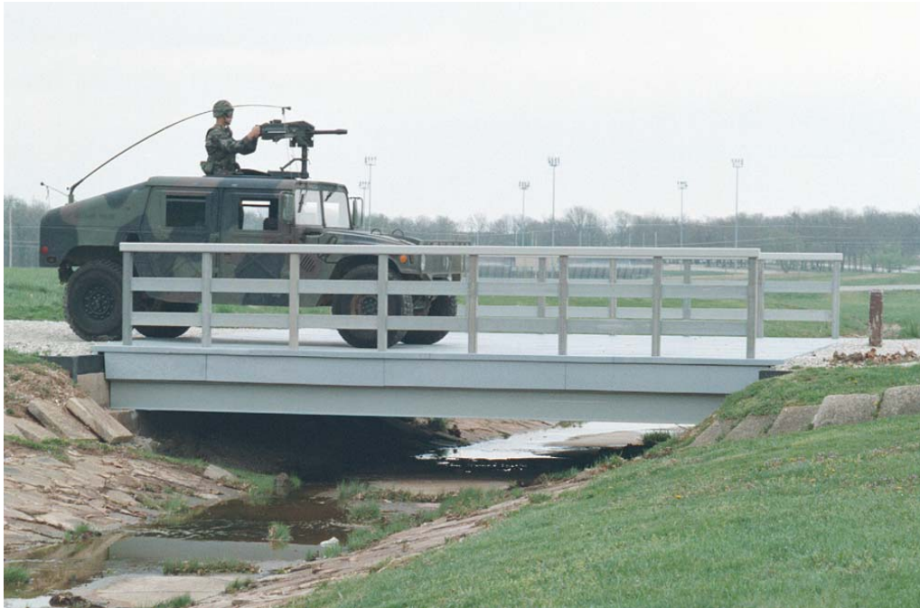
Figure 1. The first plastic lumber bridge built in the summer of 1998.
