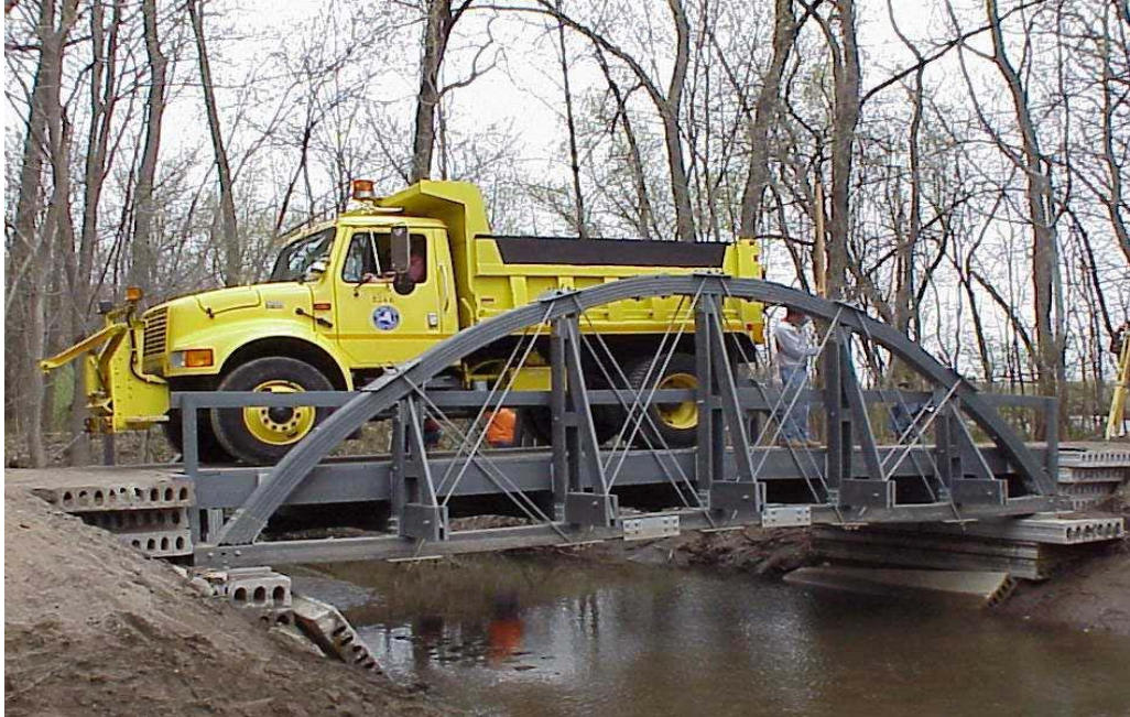
Figure 2. Load testing the plastic lumber, arch-truss bridge in Albany, NY.
