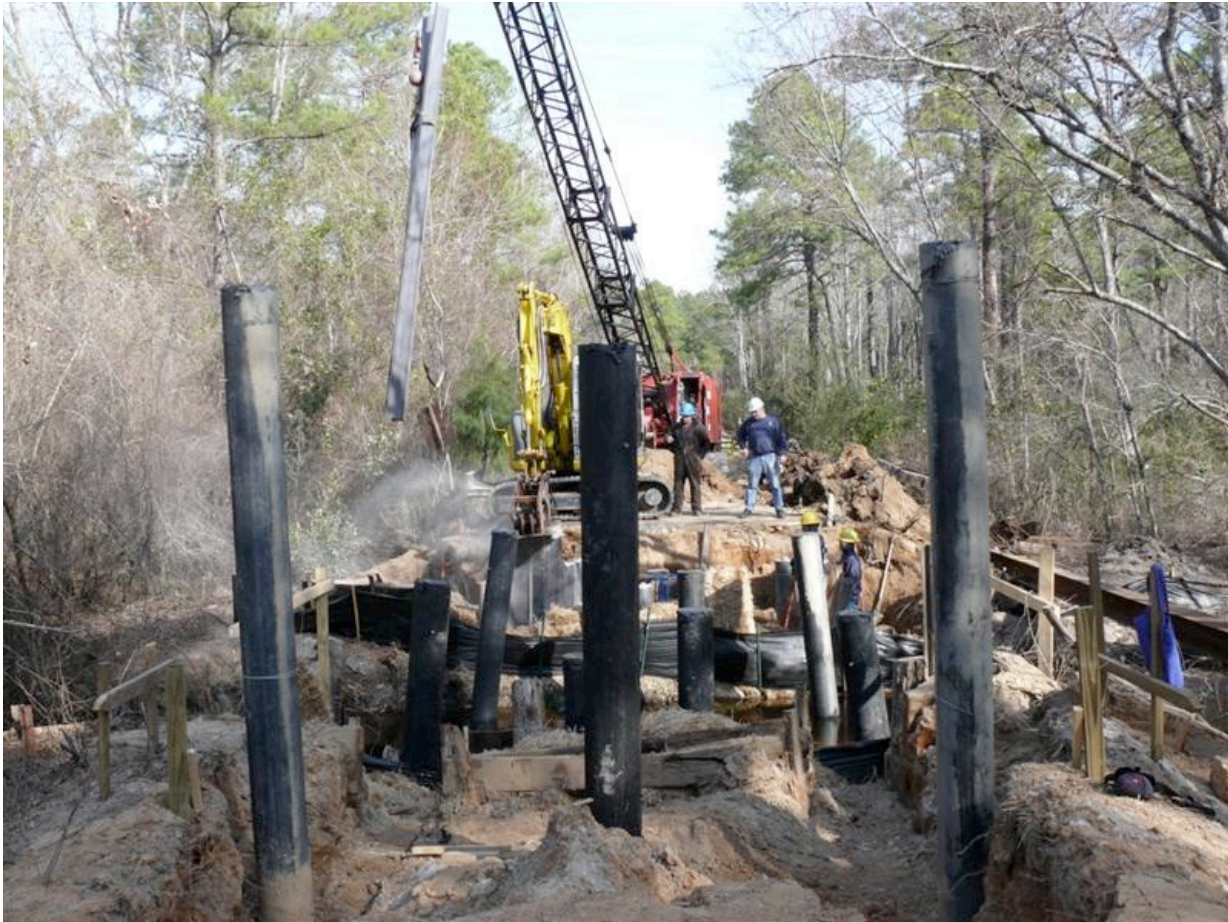
Figure 1. Thermoplastic Timber Pilings being driven at Ft. Bragg
